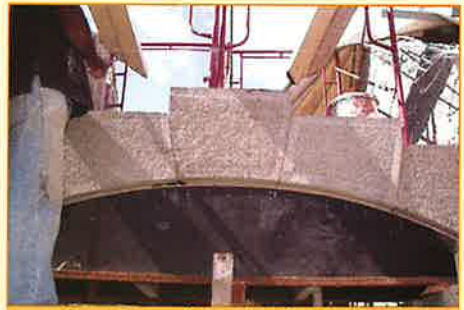
Conservation of the arch in the coach room
