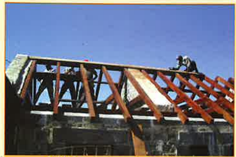
Building of wooden roof with shingles
