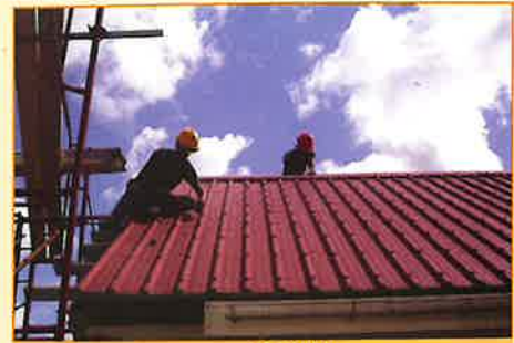
Dismantling of modern roof
