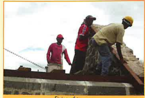
Fixing of trusses
