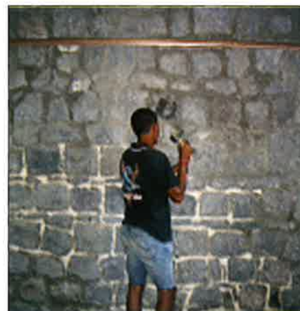
Removing Cement Pointing
