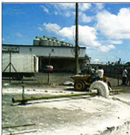
Work Yard: Grinding Lime
