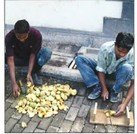
Cutting 'Bel' Fruit to prepare lime mortar
