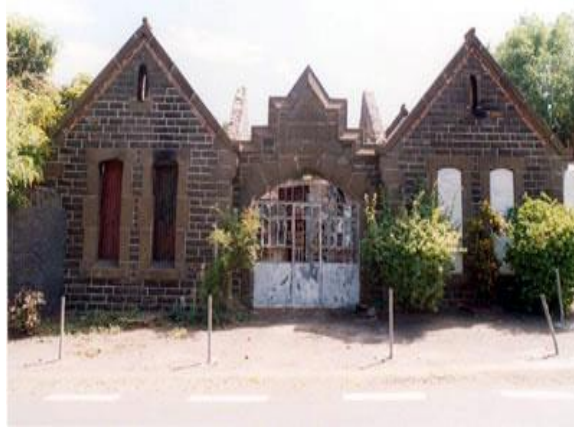
The Guard Room/Office of the Vagrant Depot was constructed between September 1866 and February 1867
