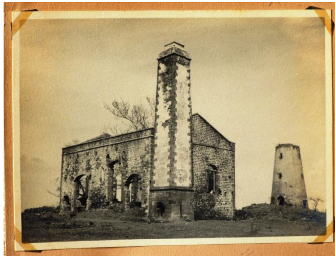
Fig 8. Overview of ruins at Forbach Sugar Mill in 1950 (Source: Mauritius Chamber of Agriculture)
