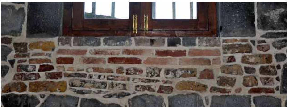
Figure 7. A variety of bricks recycled in modifications to the Surgery in Sector T. (ph 1114)
