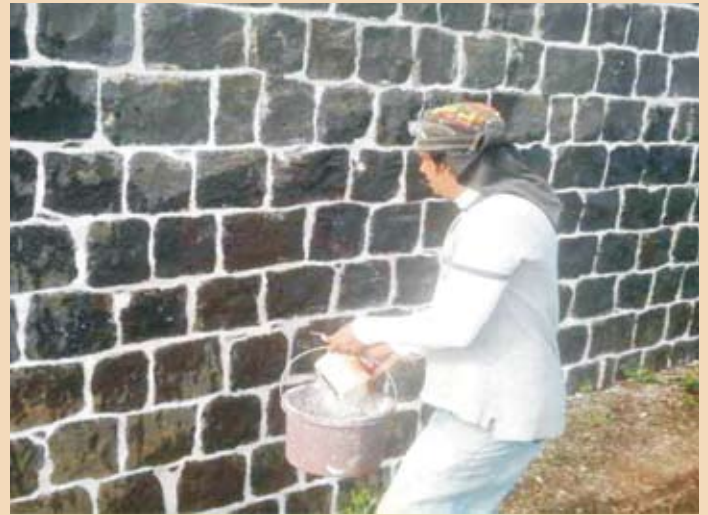
Spraying of water on repointed joints © AGTF
