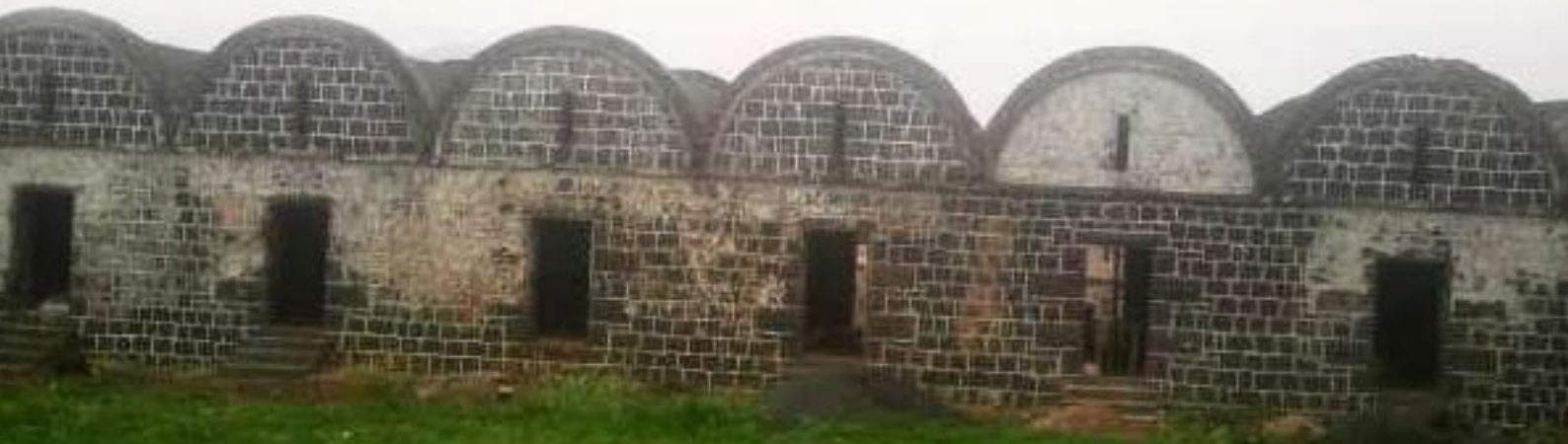
Repointed walls of the barracks © AGTF
