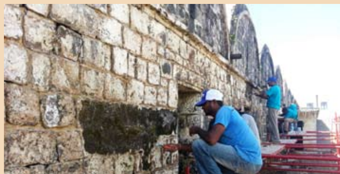
Raking of the exterior walls of the barracks © AGTF
