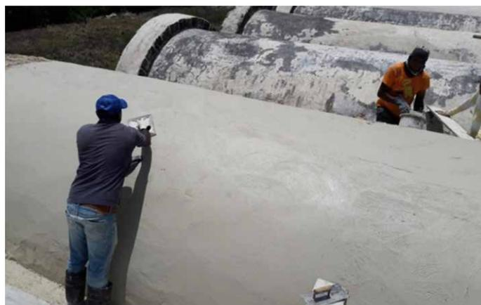
*Laying of fresh lime mortar*
