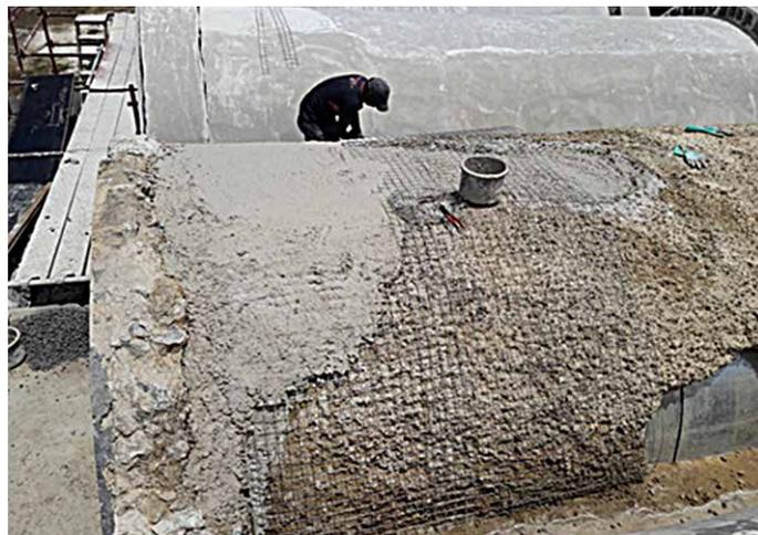
*Consolidation of roof with wire mesh*
